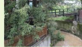
▲ Urban streams are often overwhelmed by the velocity and volume of runoff. As a result, stream banks have been engineered with concrete walls.
