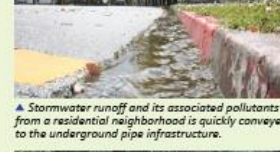
▲ Stormwater runoff and its associated pollutants from a residential neighborhood is quickly conveyed to the underground pipe infrastructure.
