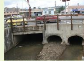
▲ Ultimately, stormwater runoff from urban conditions is carried untreated with large diameter pipes to receiving water bodies.
